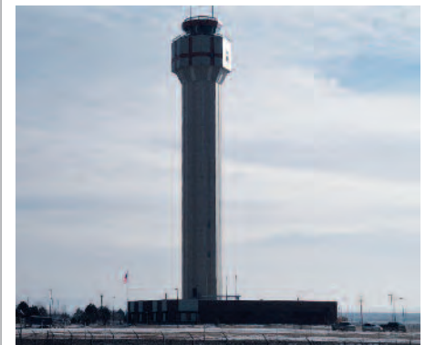
Local 291 members completed work on a new Boise Airport/FAA control tower.
